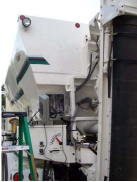
The rear of the volumetric mixer truck.
