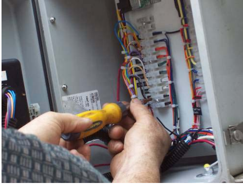
Find a free place to connect 2 wires one to the other. If there is no label, stick a label in order to remember that these wires command the fiber feeder.
