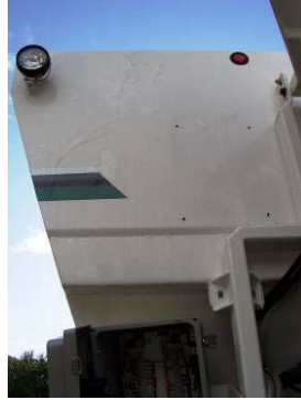
Bore 4 holes in the rear wall (the cement tank in that case)
