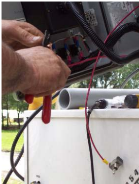
Find a free place to connect 2 wires one to the other. If there is no label, stick a label in order to remember that these wires command the fiber feeder.
