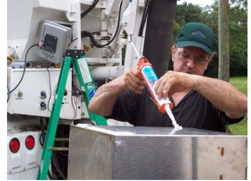
Add some sealant around the holes to prevent rain water to blow in the box.
